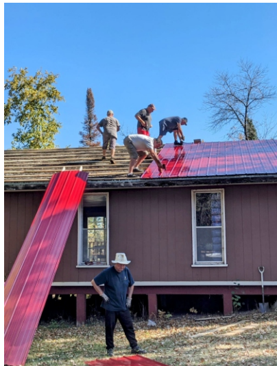
Renovation work continues at Camp Copernicus!
